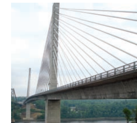
The Penobscot Narrows Bridge, Maine's first cable-stayed long-span highway bridge, opened in December 2006. In June 2007, Lawrence Tech collaborated with the Maine Department of Transportation, the Federal Highway Administration, and Figg Bridge Engineers to replace six strands with carbon fiber composite cables – a first in the United States. These strands are being monitored in order to evaluate this material for future use in bridge designs.
