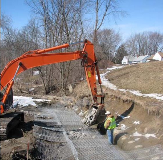
The installation of the gabion baskets was completed with heavy machinery. (Picture—M. Best)
