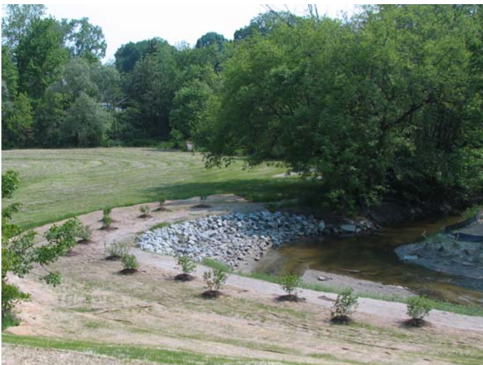
The finished bank with added floodplain storage shelf. (Picture—M. Best)
