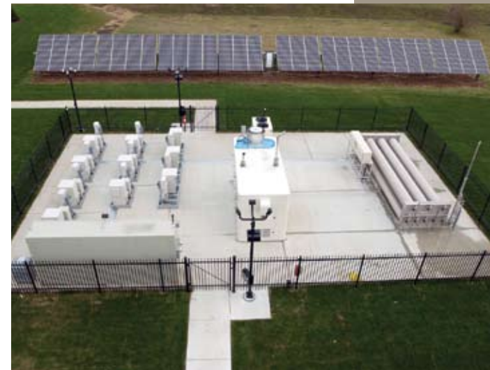
Lawrence Tech is the educational partner for the DTE Energy Hydrogen Park in Southfield, the first and largest hydrogen technology park of its type in the world. It was developed with support from the U.S. Department of Energy. Lawrence Tech faculty and students have helped research the use of hydrogen for both electricity and transportation fuel.
