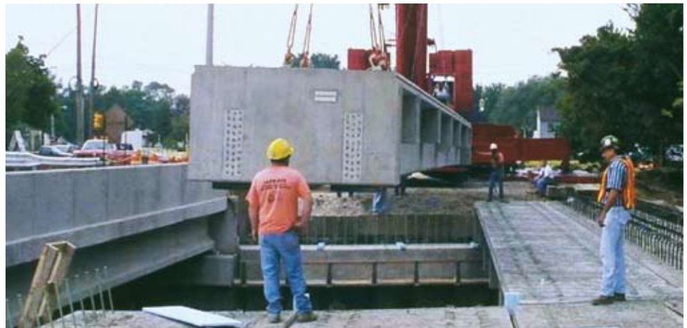
This three-span bridge was designed with precast concrete components incorporating carbon fibers about the diameter of a human hair that are woven together and encased in epoxy. The design offers key advantages over steel strands, and those benefits will be tested via monitors on the bridge.
