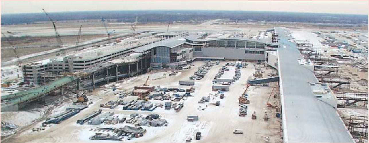
Overview of construction of parking structure. Photograph was taken December 5, 2000.
